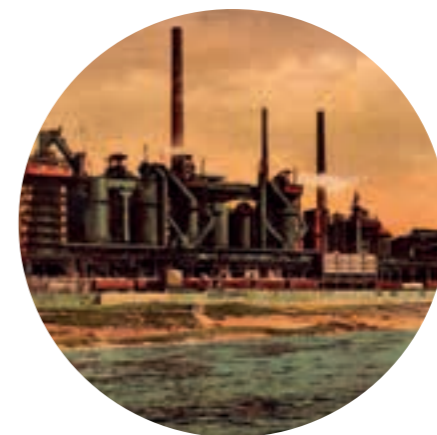
The transition to the hot blast process marked a new stage in the history of blast furnace design
